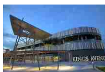
2 KINGS AVENUE MALL
