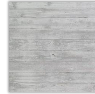
Horizontal board frame concrete (External walls)
