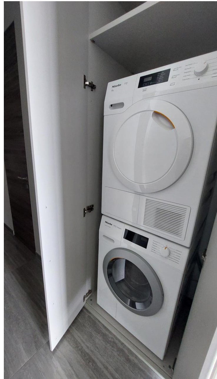
DRYER / WASHING MACHINE
